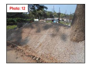
Excavated earth has been stacked irregularly and haphazardly. Advised to immediately to remove the garbage waste from construction site (Photo: 13).
